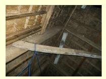
With the scaffolding in place it provided access to the old electrical cabling that is being removed. It is being replaced by a new electric cabling infrastructure to modern standards and requirements. The new electrical circuits have to be installed before the insulation is added and plasterboards can be fixed.
