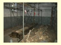
The battens in the hall ready to be moved onto the scaffolding in readiness for fixing. As the existing rafters are oak stainless steel screws are required to fix the battens.
